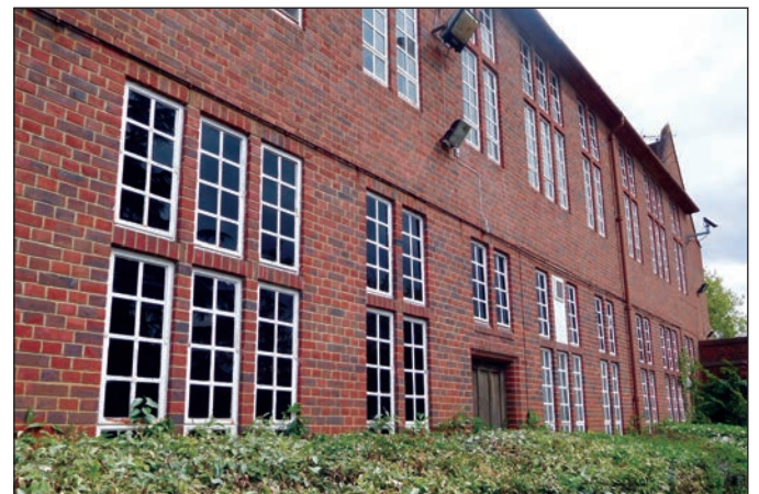
More red brickwork – and windows.
