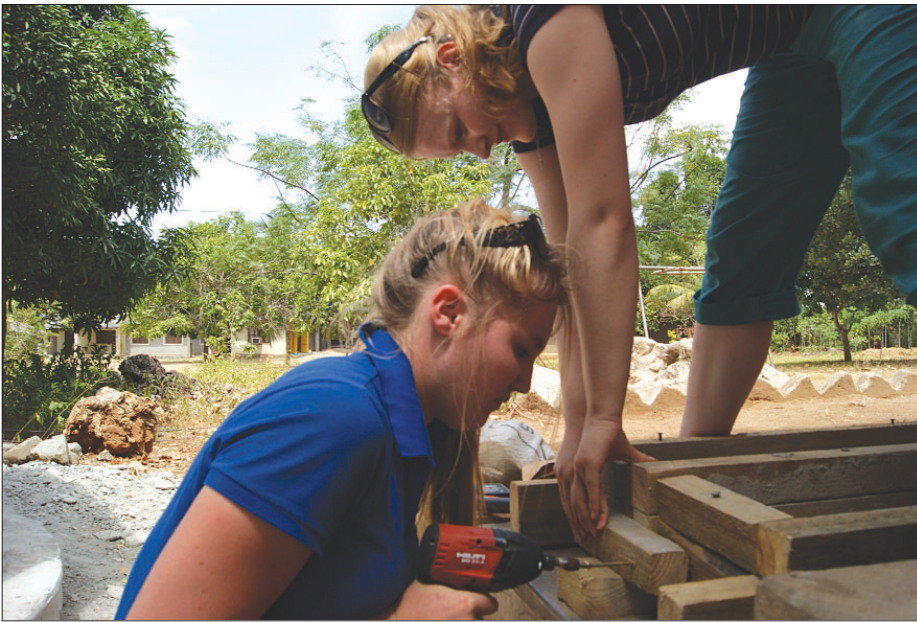
Fixing the roof
